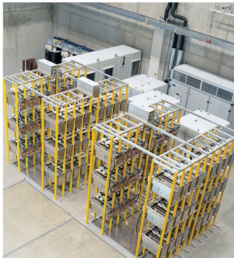
Modular multi-level converter.
